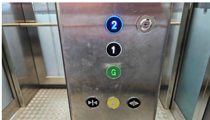
Controls in the main lift. Note: raised features.
