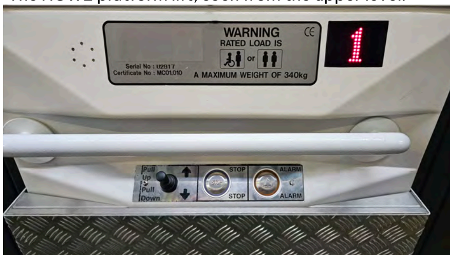
The platform lift controls. Note joystick and alarm button.
